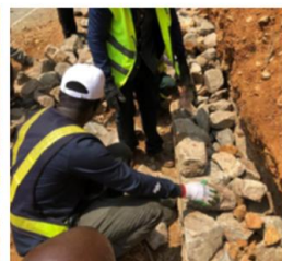
Figure 7: Construction of dry-stone toe wall
