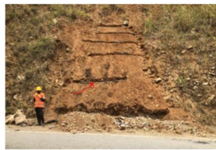
Figure 4: Installed Fascines
