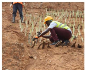
Figure 5: Installation of grass and brush layers
