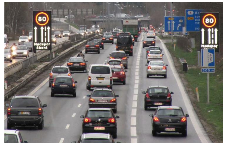
Hilleroad motorway, Danemark
